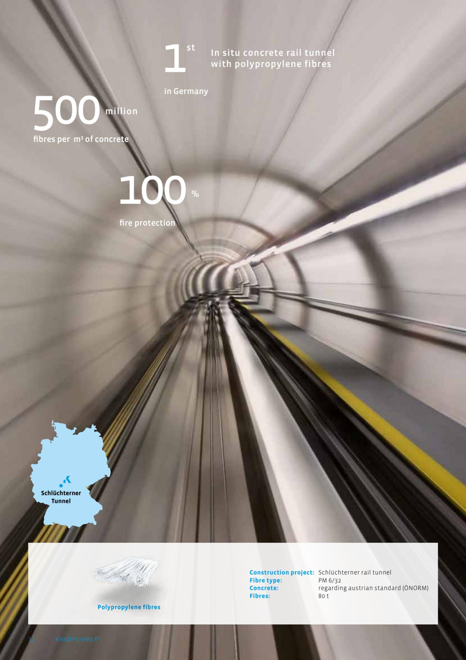
**1<sup>st</sup>** In situ concrete rail tunnel with polypropylene fibres in Germany
