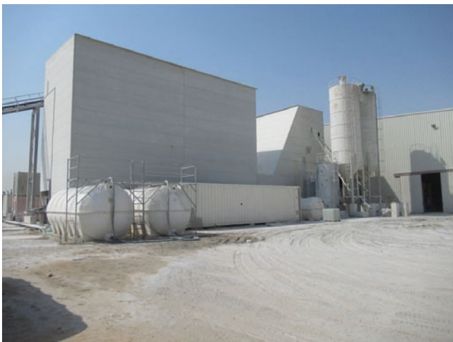
Batching Plant, right side
