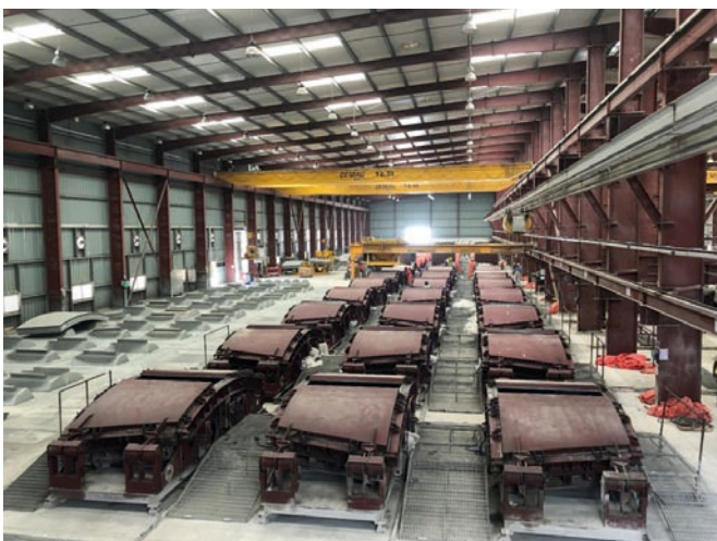
Precast Segment Factory, left side
