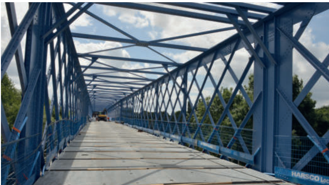
The Mauves-sur-Loire bridge consists of UHPFRC precast elements which have been made at Delta Prefabrication plant located in Privas (France). In this project, the fibers used were 14 mm / 0.2 mm steel brass coated. Joints were poured with ultra-high-performance fibre-reinforce concrete.
