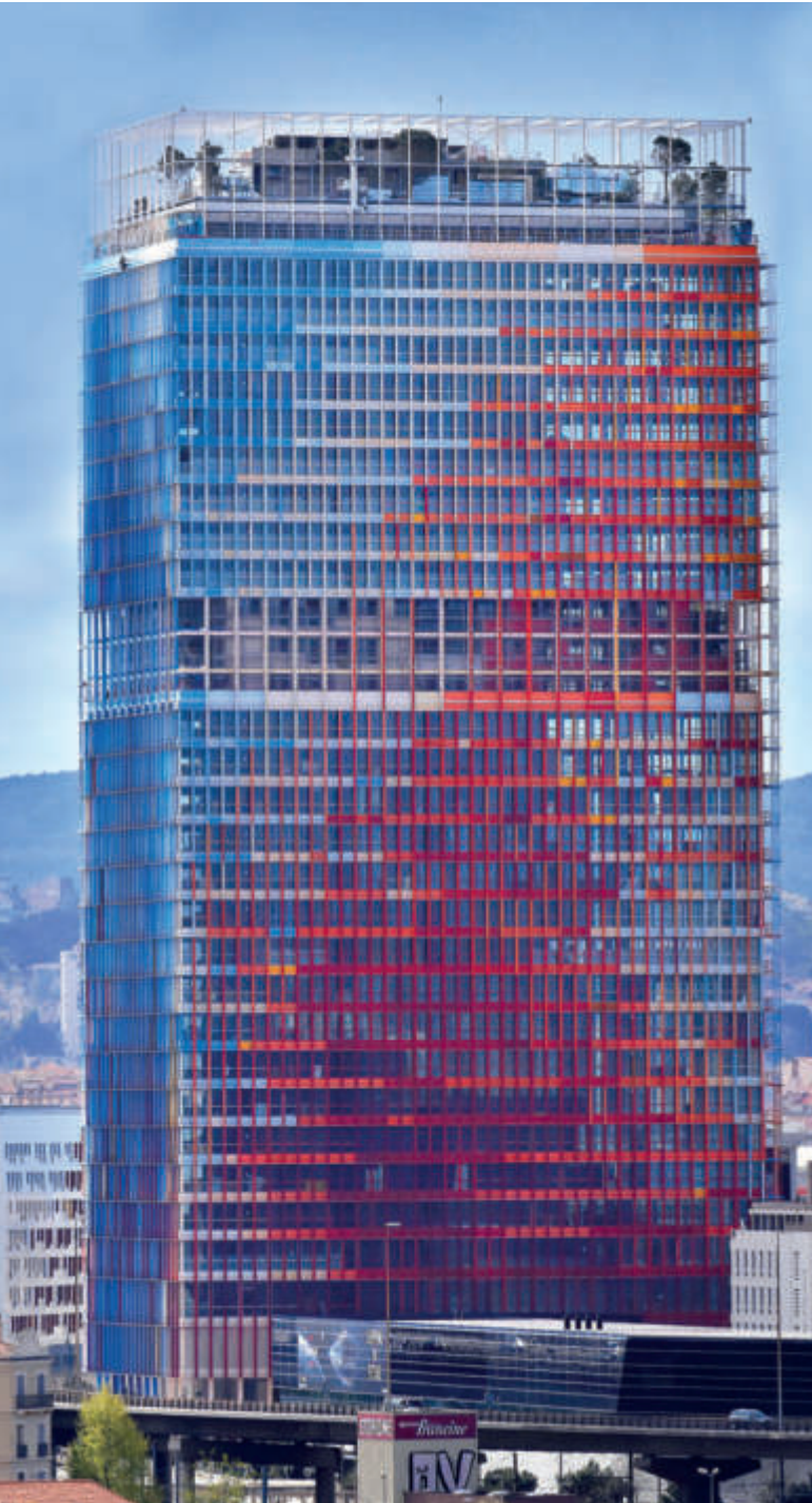
Marseille’s new high-rise tower façades are composed of Ductal prefabricated elements that participate in the building envelope’s thermal insulation, solar control, building maintenance and fire partitioning.
