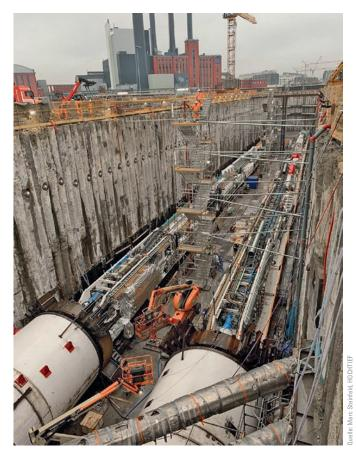
Bild 2 TBM "Inge" und "Olivia" im Startschacht Enghave Brygge (EBR) TBM "Inge" and "Olivia" in the starting shaft Enghave Brygge (EBR)
